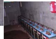
PNT-907 Battery Room W/ 60 Batteries
