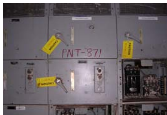
PNT-871 Motor Control Center
