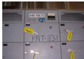
PNT-831 Motor Control Center
