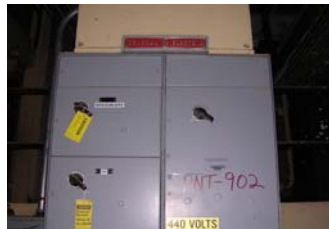
PNT-902 Motor Control Center
