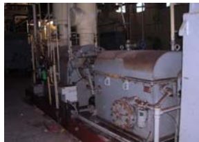
PNT-869 Pump & Motor Assembly
